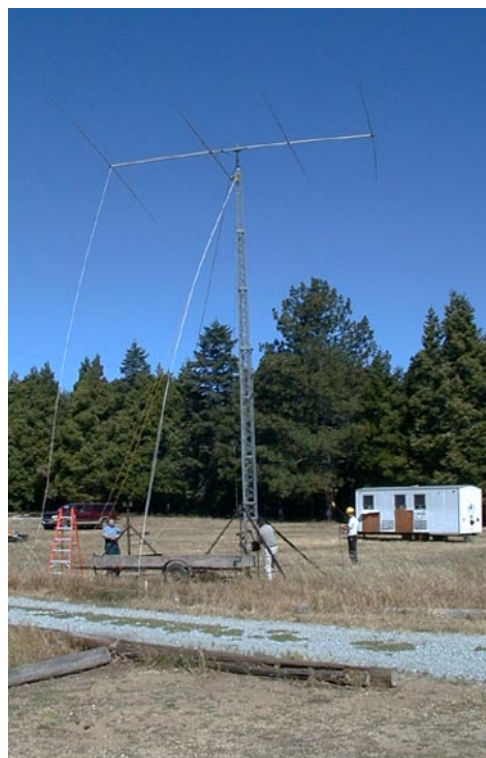
15 meter portable tower
